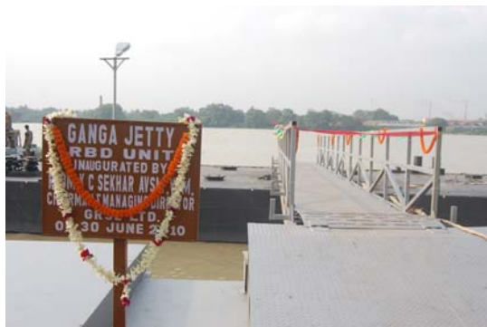
Jetty decked up for commissioning
